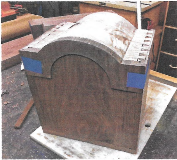
The initial fitting of the door panel. The gap at the top of the door was narrowed by the addition of a thin strip of walnut to the door.
